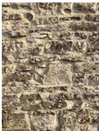
Natural rubble stone wall with lime mortar pointing
