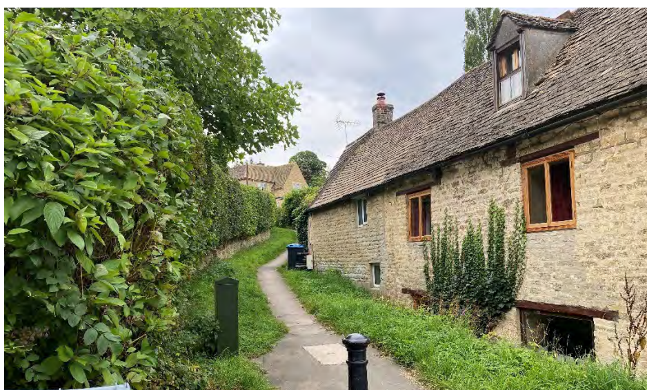
Figure 19: Looking up Well lane, timber lintels, houses backing on to routes, low roof with slate finish easily visible as buildings address change in ground level.
