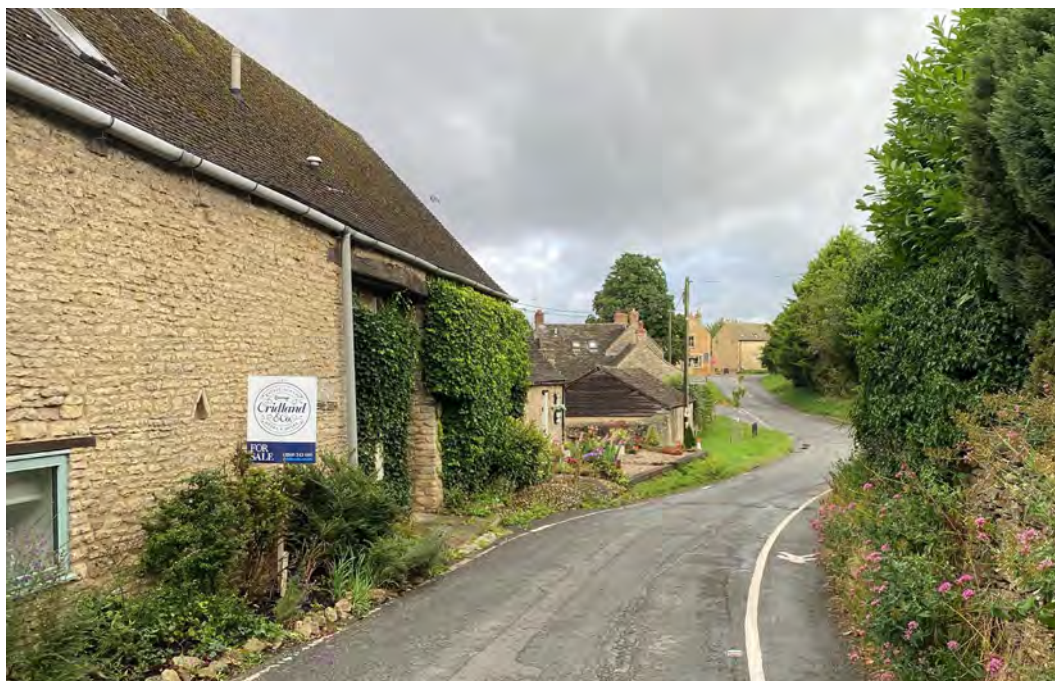
Figure 38: view from Pond Hill towards the White Horse past converted former farm buildings and over the Green.
