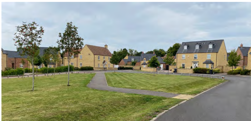
Figure 50: William Buckland Way where red clay tiles, blanket use of Welsh slate, and red brick walling are starkly in contrast to the local vernacular.
