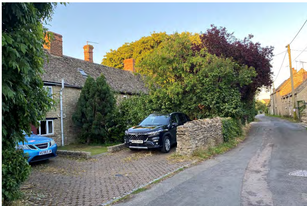
Figure 12: Loss of dry stone wall and provision of atypical red brick surfacing to provide parking, though beneficial to remove parking from the narrow street.
