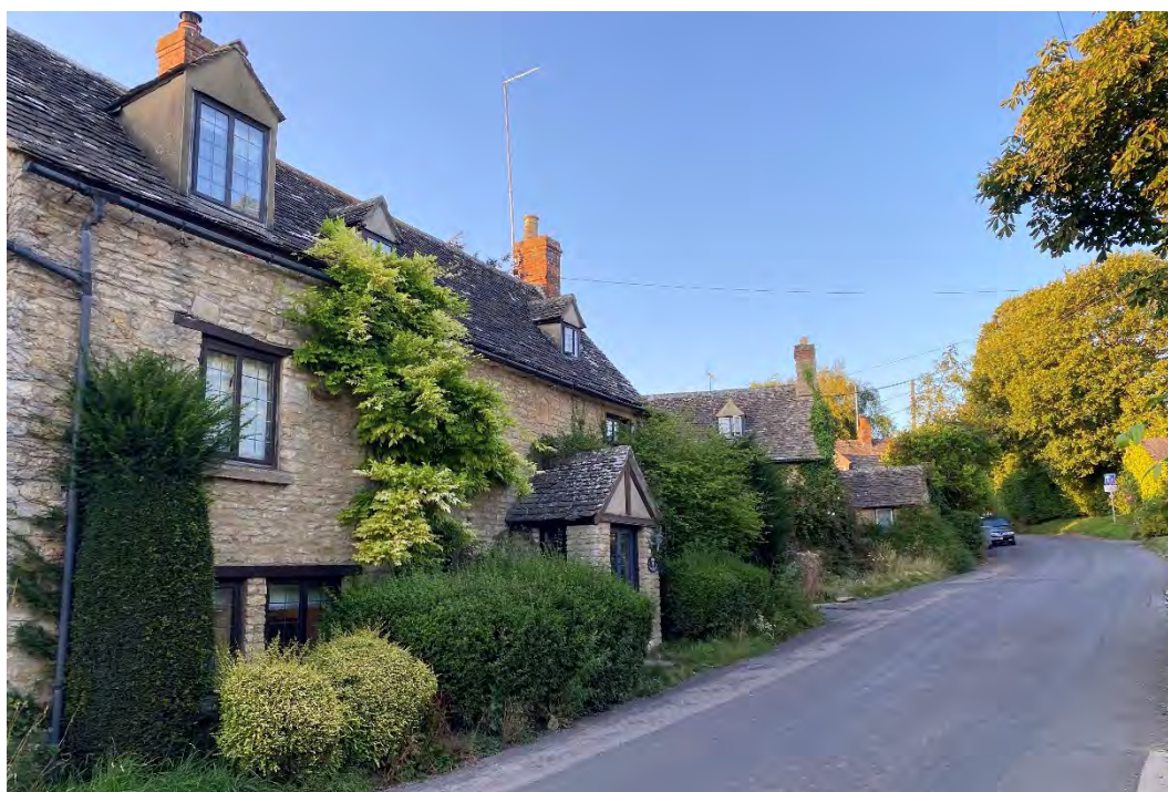
Figure 20: Building line close to the road, timber lintels, wooden casements – here modern leaded replacements – an added porch and gabled dormers with brick chimneys, many of the characteristic features found in the historic core of the village.
