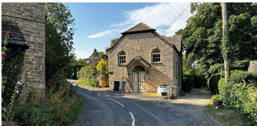
Figure 14: Converted Wesleyan Methodist chapel then Sunday school, where former religious use remains legible in the style of openings. The building has a half hipped gable end, an unusual form within the village.
