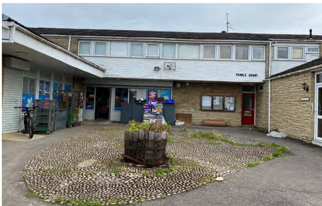
Figure 48: Pendle Court shops
