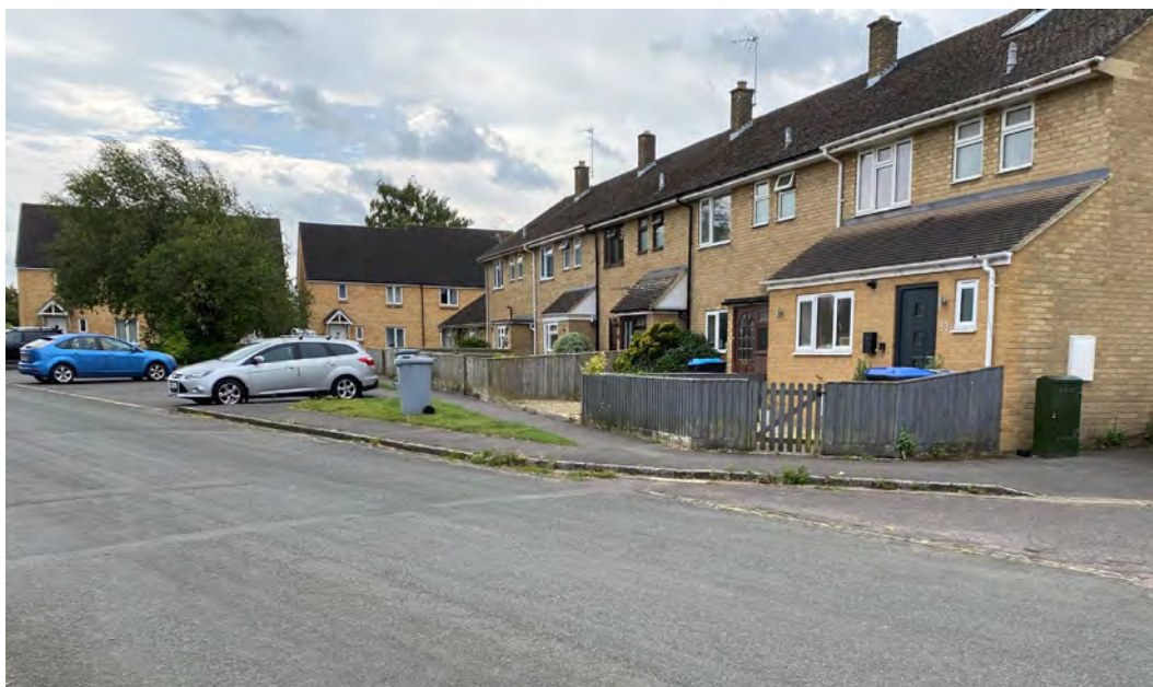
Figure 51: terrace on Longore set back to create a triangle of open grass by parking and marked with trees.
