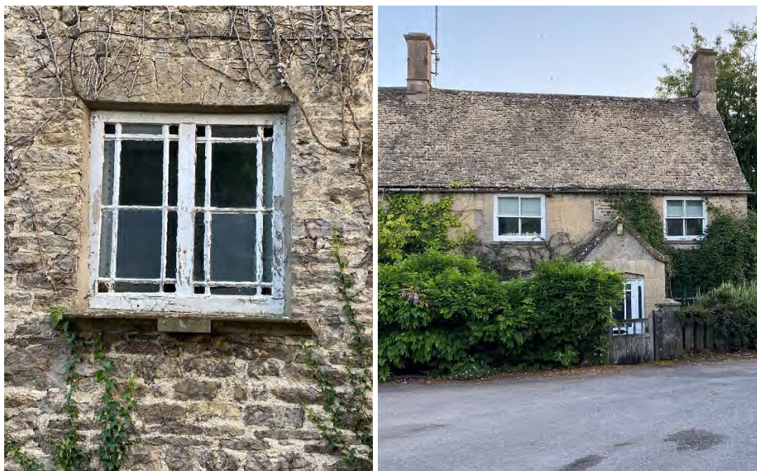
Figure 21-22: An unusual example of a window with narrow margin lights and stone splayed window head and dressed sill, on The High Street, part of Austin's Farm (left) and, 2/2 sash windows on Protestant House on The Cross (right), which also shows comparatively rare render finish to the walls.
