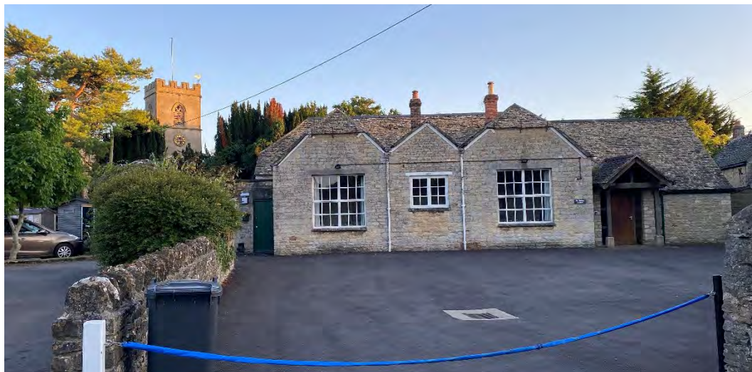
Figure 17: The Victorian school building, and tower of St James behind. Note use of half hips, unusual within the village.
