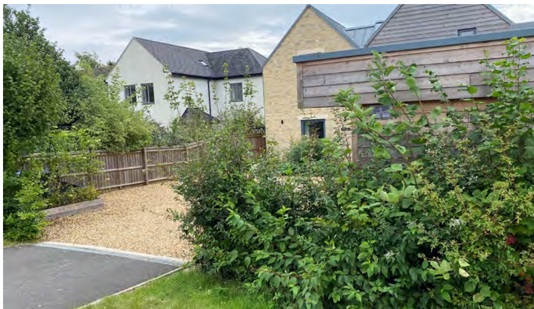
Figure 46: More recent houses incorporating alternate materials on Woodstock Road.
