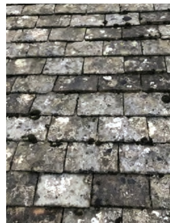
Plain grey concrete tiles with lichen and moss
