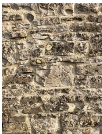
Natural rubble stone wall with lime mortar pointing
